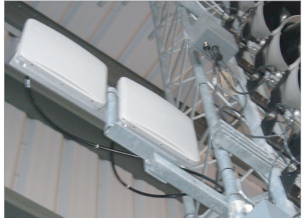
RFID antennas at the Brampton Intermodal Terminal
